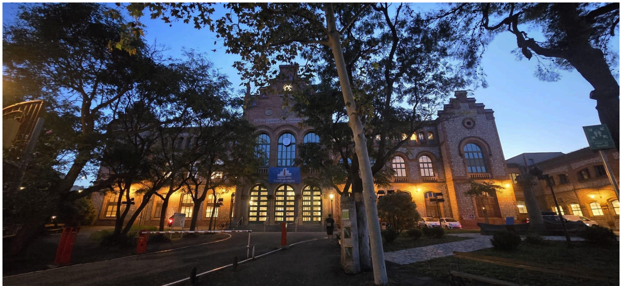
Photograph 1. Facade of the TR-1 building
