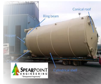
Stiffness of a silo superstructure
